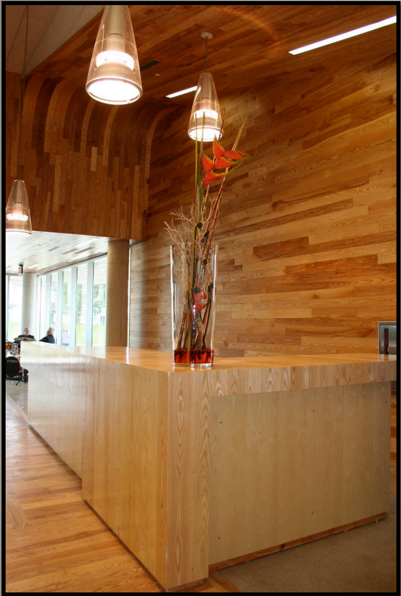
Traverwood Branch of the Ann Arbor, MI library. Ash trees removed from the new branch library site were incorporated into the building's construction as support beams, flooring, and shelving.
